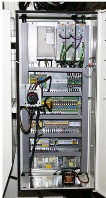
EVS-760B CNC ELECTRICAL CABINET
